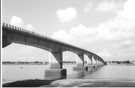
Kompong Cham the Japanese Bridge across the Mekong
