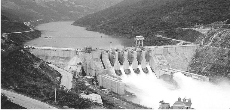
Dachaosan 1,350 MW: the second mainstream dam in the Mekong Cascades, started in 1996 and completed in 2003 [source: Tom Fawthrop]
