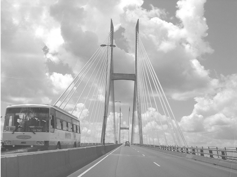
Crossing Mỹ Thuận Bridge, a cable-stayed bridge over the Tiền River.
