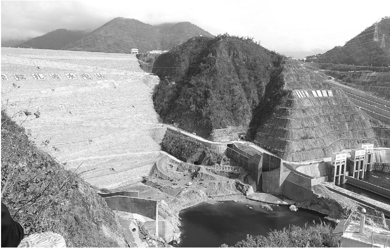
Nuozhadu 5,850 MW, the sixth and the largest hydroelectric dam on the Mekong River, started in 2006 and completed in 2014. The white letters on the right: “Power comes from water – Ability to contain generates great things” [source: Ying Qiu, International Rivers]
