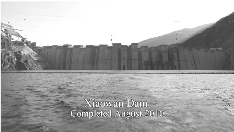
Xiaowan Dam 4,200 MW: the fifth and the tallest mainstream dam in the Mekong Cascades, started in 2001 and completed in 2010 [source: Tom Fawthrop]
