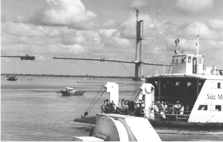
Mỹ Thuận Bridge 11.1999 near completion
